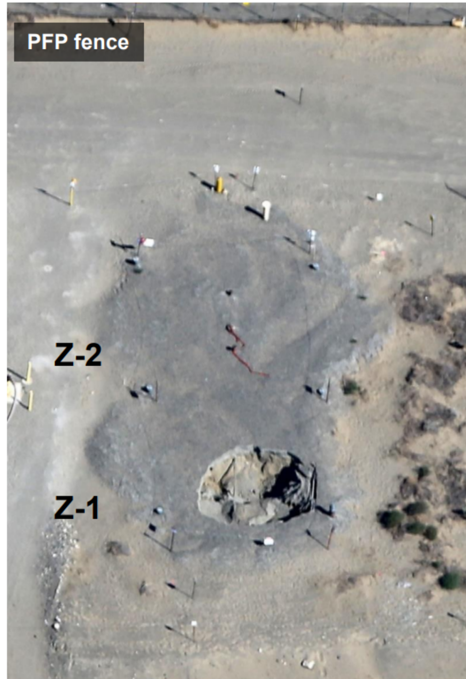
Photo taken in (2016). Subsidence over Z-1 has been backfilled.
