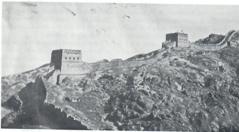
Figure 4. The Great Wall, China. Although it has stood for twenty centuries, the Wall has required continual maintenance, something the marking system for the disposal sites must avoid. One-piece construction for each component would minimize this problem.
