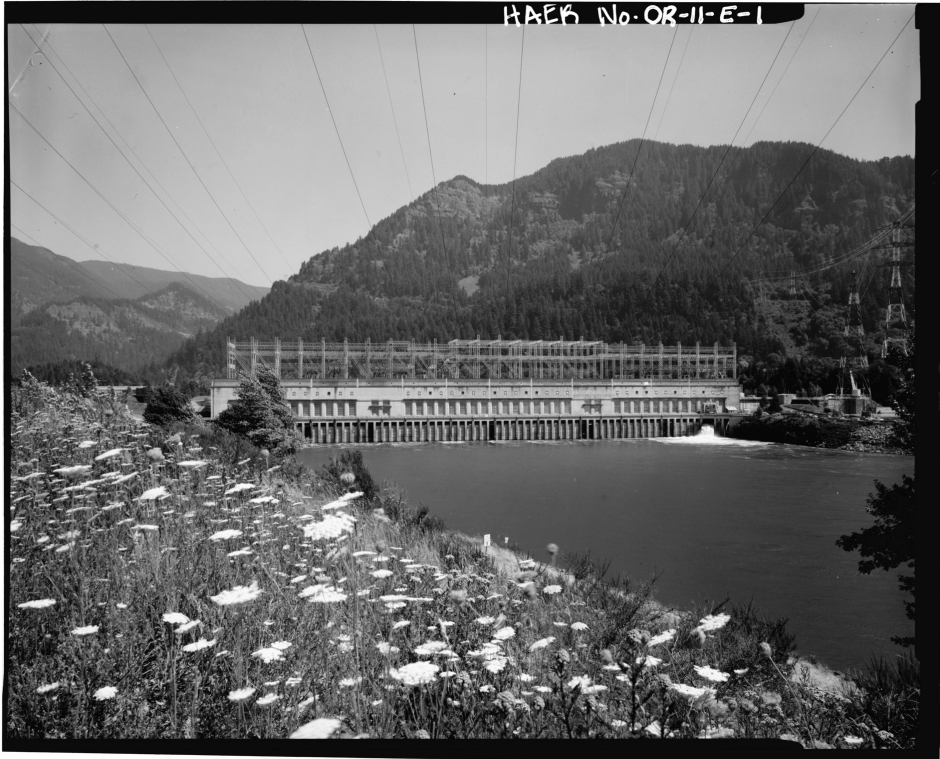
Fig. 5: Downstream Face of Powerhouse One (from Bradford Island). National Parks Service.
