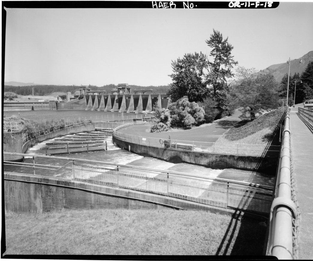
Fig. 9: Bonneville Dam, Bradford Island Fish Ladder. National Parks Service.
