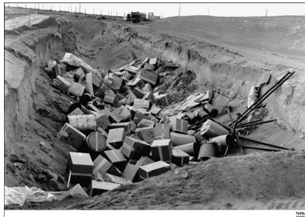
Fig. 9. Poorly characterized radioactive and non-radioactive solid waste was buried onsite during the early years of Hanford (US Department of Energy).
