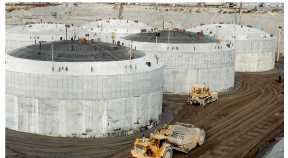
Tanks under construction Image courtesy of USDOE
