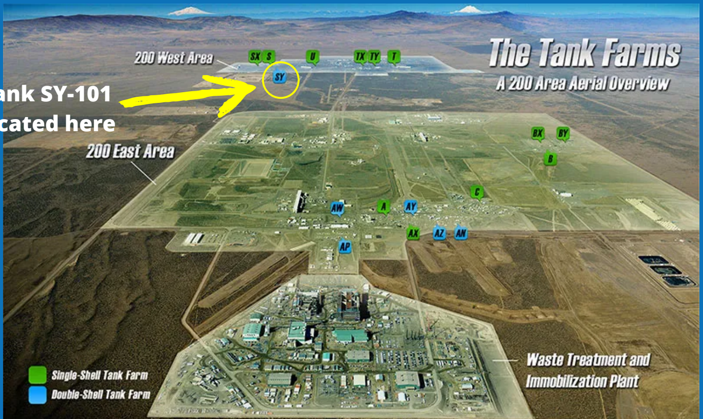
Aerial view of Hanford's tank farms and Waste Treatment and Immobilization Plant. Image courtesy Washington River Protection Solutions
