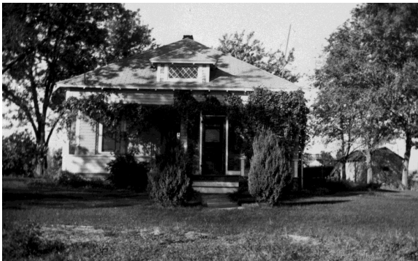
House, White Bluffs, 1940. Photo: U.S. Department of Energy
