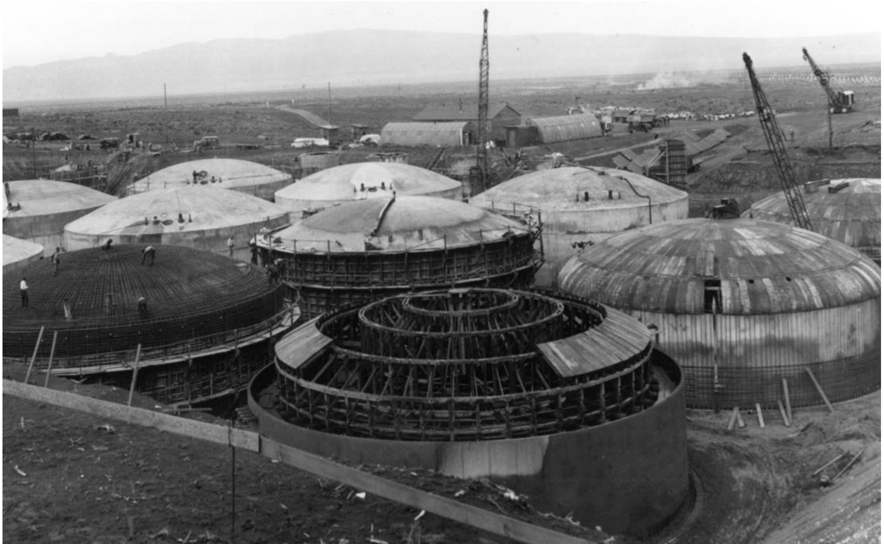
Hanford Underground Tanks Construction
